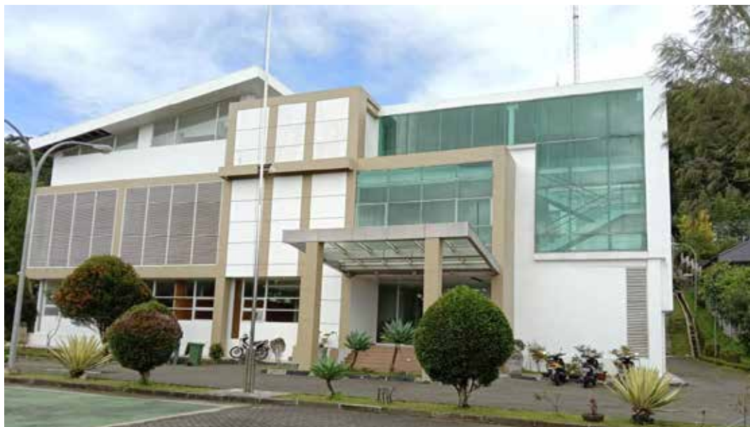
Foto Gedung Arsip PPATK, Ciloto, 2020. Photo of PPATK Archive Building, Ciloto, 2020.
